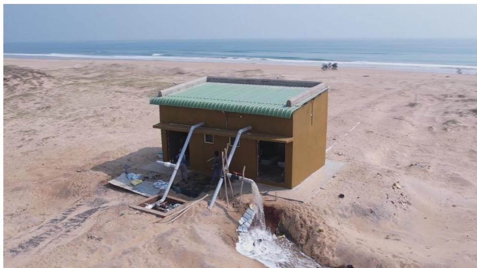
**3. Main Water Supply Line:** The water from the pump house will be carried over a distance of nearly 500 m through a set of pipelines to the reservoir ponds and to the primary circular reservoir separately but could be redirected to one another by a control system
