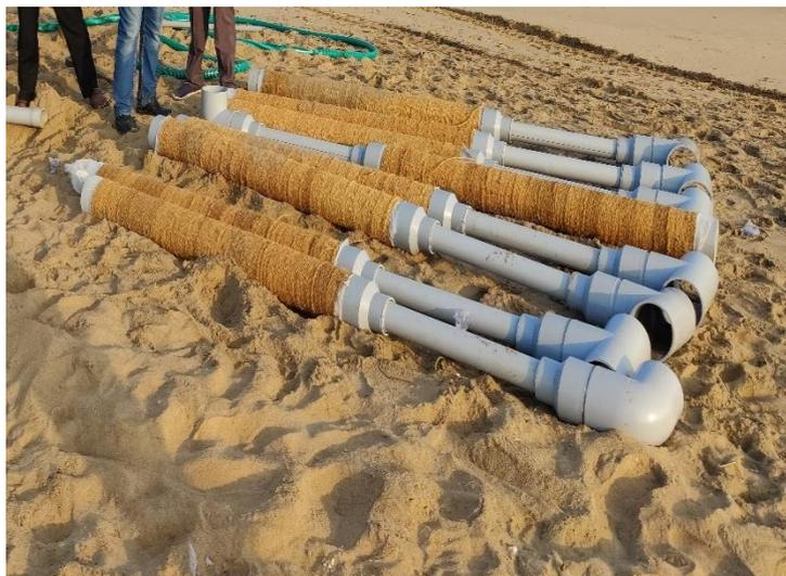
primary reservoir. The beach bore well system is designed for 150m<sup>3</sup> per hour supply to the primary reservoir.
